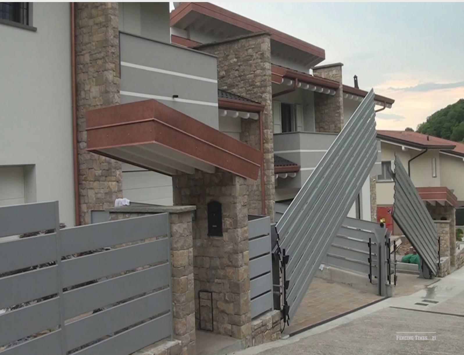
**T**he main difference with the 1 series is the drive pillar. In the 1 series the controls and other electronics were housed in a separate cabinet, installed up against the pillar. "Now we have a gate column which contains and accommodates both the hydraulics and the electronics," CEO Loris Gentili says.
