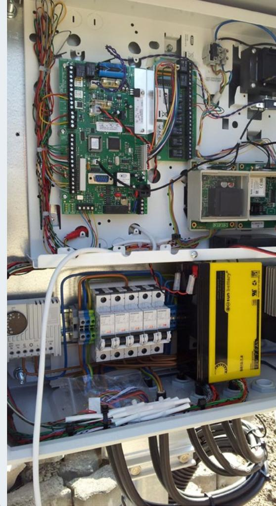
Field cabinet with power supply, emergency power supply, burglar alarm control panel with alerts via the mobile network, and a heater with a thermostat.
