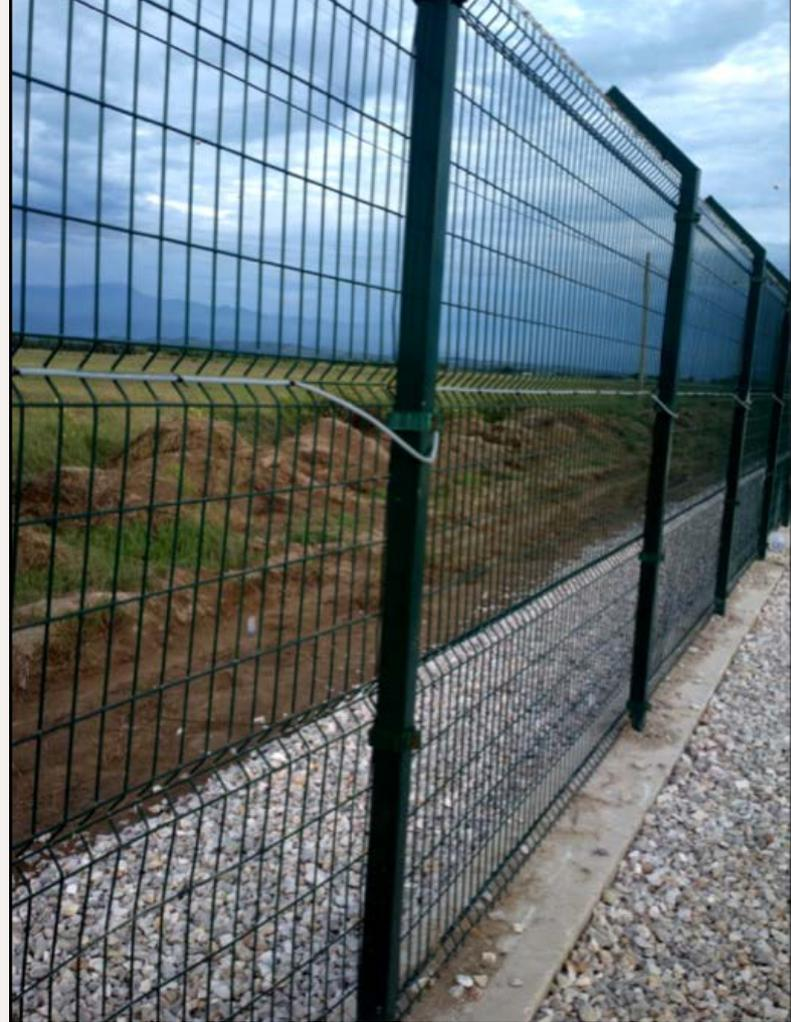
Here, the fibre-optic cable is attached to the 3D bend of the single wire panel. Don't forget the gravel strip; it ensures that there is no vegetation to blow around and cause vibrations in the fence in windy conditions.
