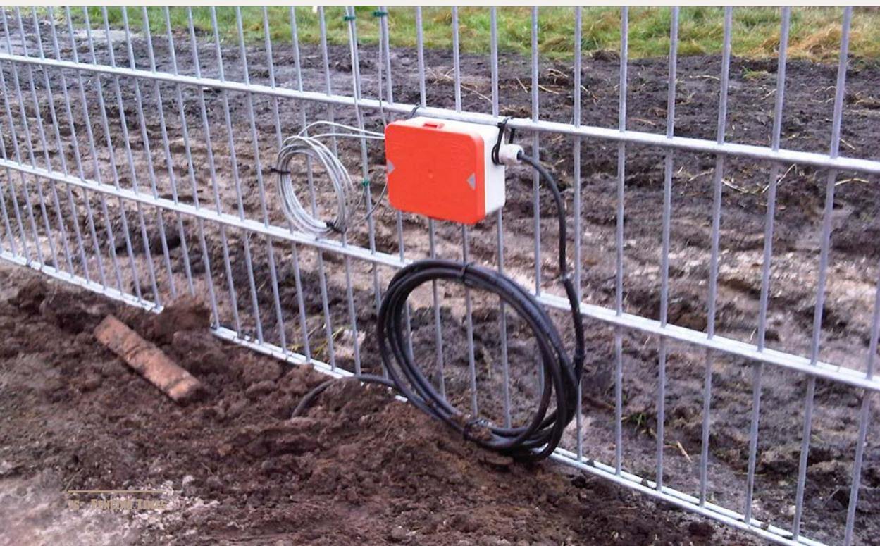
Here you can see the weld between the insensitive (black) cable and the sensitive (white) cable on the fence. Both cables are installed with a certain amount of excess length so there is enough available if repairs are required.
